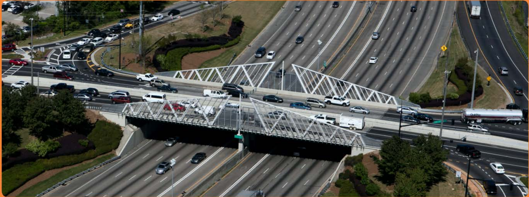
New Diverging Diamond Interchange Bridge at Jimmy Carter Boulevard
